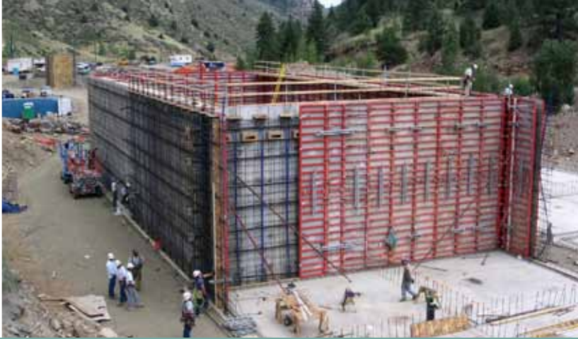
▲ Formwork construction prior to concrete placement
