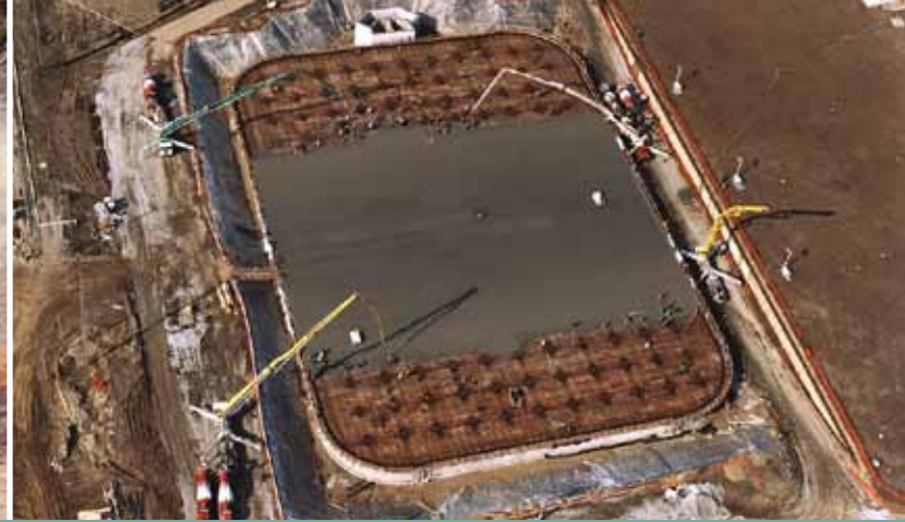
▲ Placement of roof slab concrete 2
