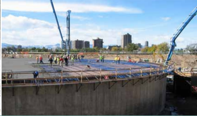
▲ Placement of roof slab concrete 1
