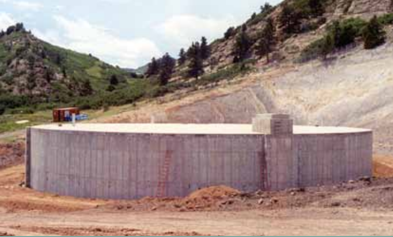
▲ Completed tank structure prior to burial 1
