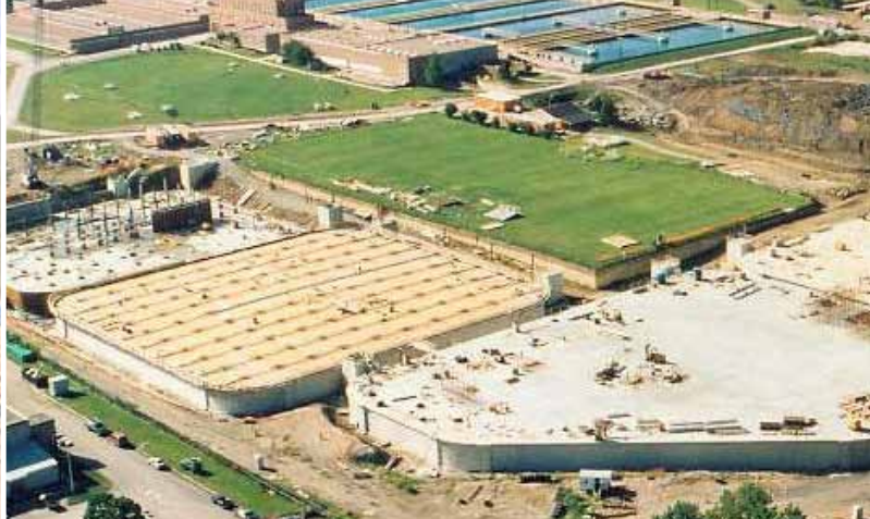
▲ Uniquely shaped post-tensioned tanks under construction 2
