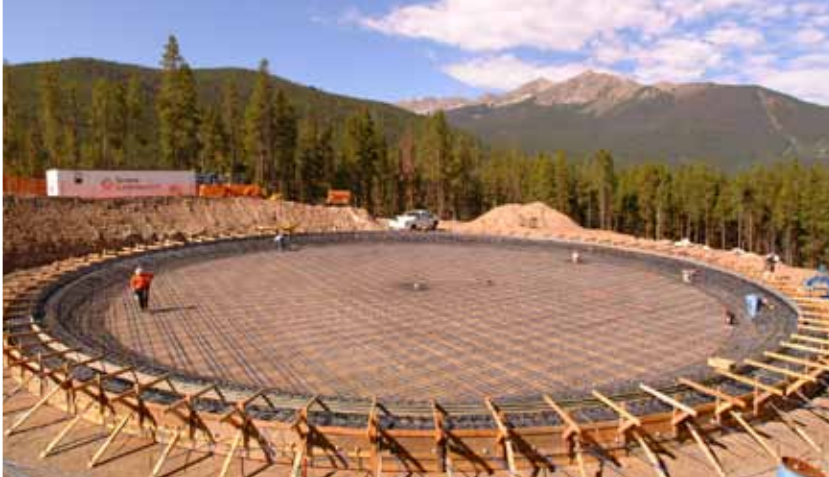
▲ Floor post-tensioning and formwork prior to concrete placement 1
